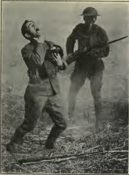
FIG. 5.—The Defective Gas Mask.
